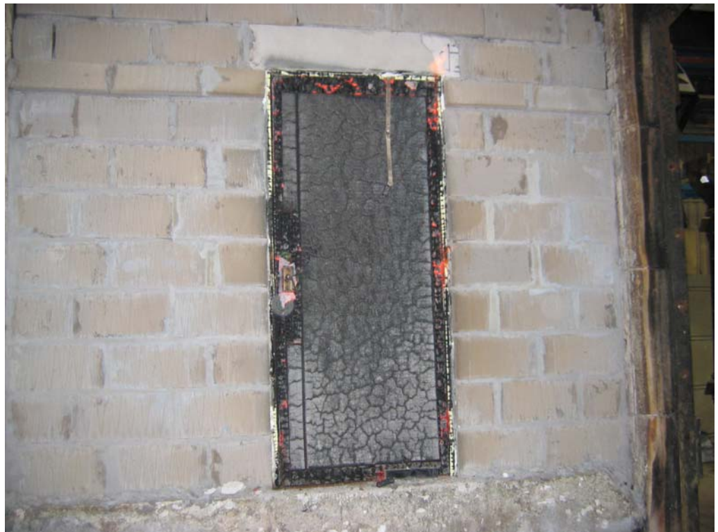
The exposed face of the test construction immediately after the test
